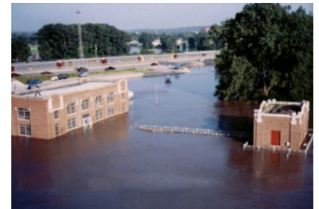
The Kansas City, Missouri, Water Treatment Plant during the flood of 1993.
