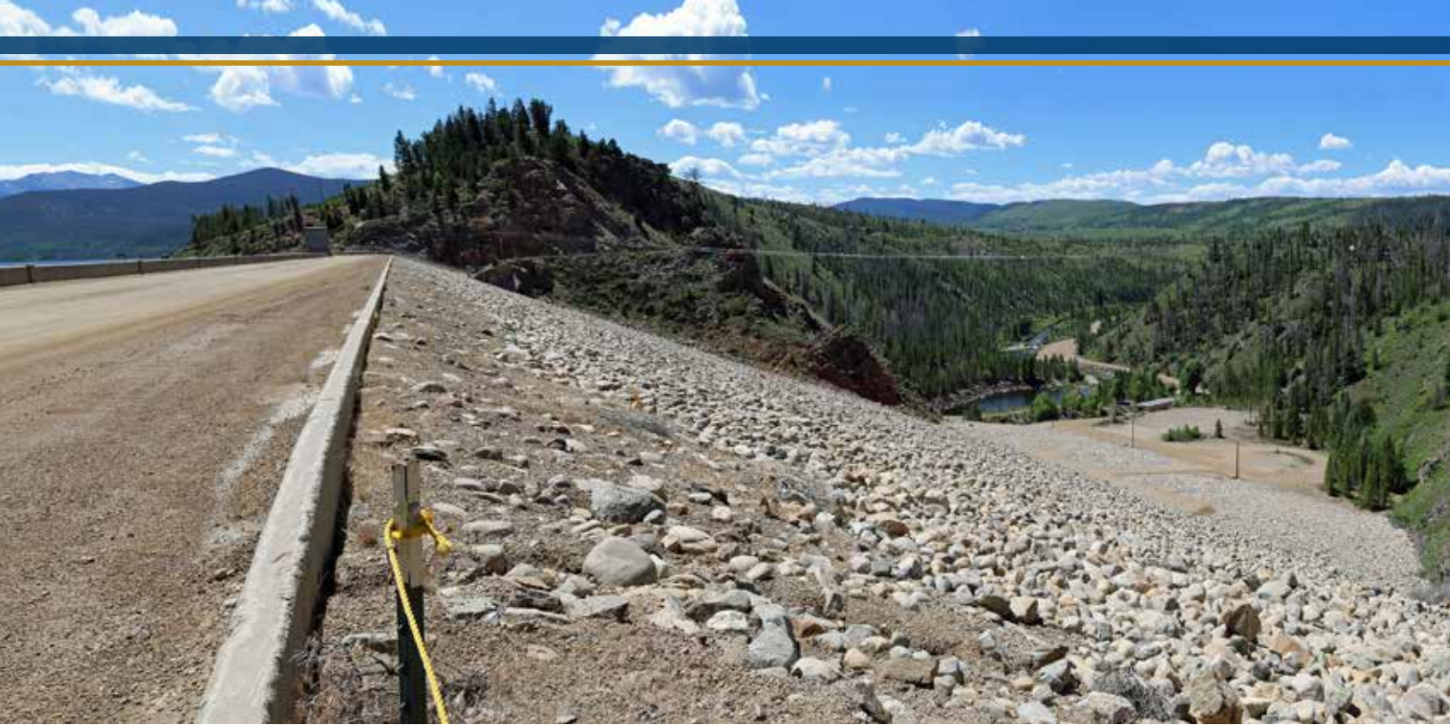
Granby Dam in Grand County, Colorado. Photo: Jeffrey Beall, Wikimedia Commons.
